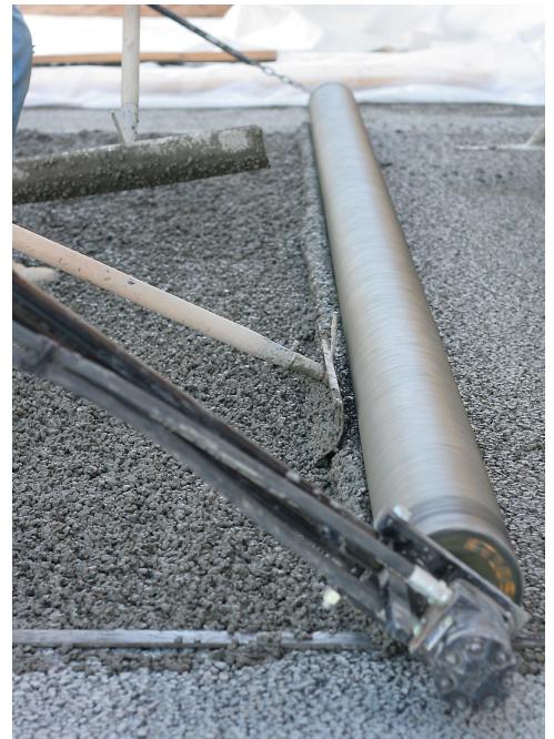
Striking off the pervious concrete with a special hydraulic roller-screed
